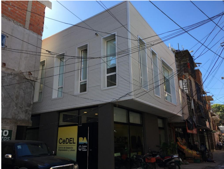
Figure 1: EDGE certified office building in Barrio 31, Buenos Aires
