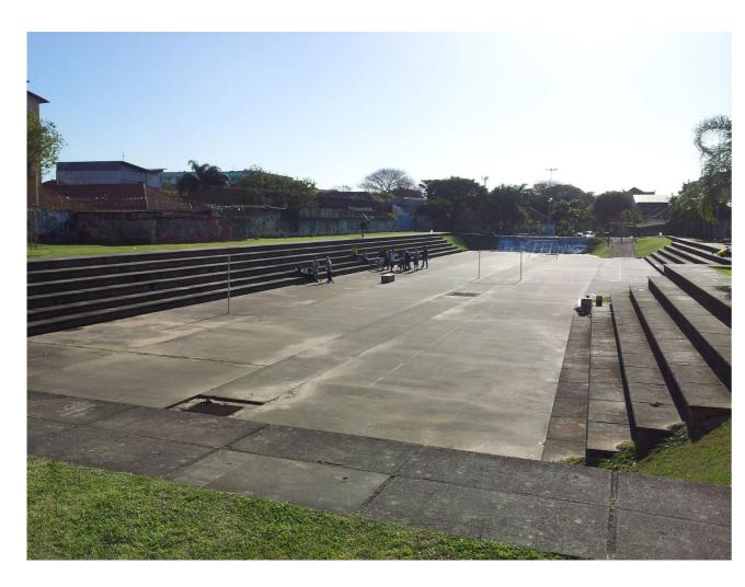
Figure 23 Detention basin in Porto Alegre with an impermeable bottom, used when there is a risk of groundwater contamination due to high pollutant loads (Photo: Erika Tominaga, 2023).
