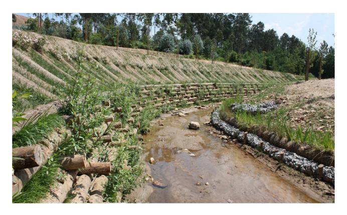
Figure 50 On the left bank, wooden cribwall with a double layer planted with native shrubs and live bundles, coconut biomat, and hydroseeding; on the right, cylindrical gabion filled with stones and vegetated coconut bio-retainer, Ribeira de Gende, Portugal (Project by Rita Sousa, photo: Rita Sousa, 2011).
