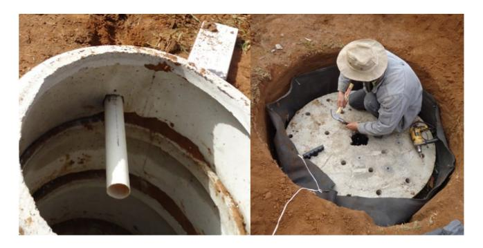
Figure 21 Infiltration pit (Source: Thays Santos Ferreira, 2018).
