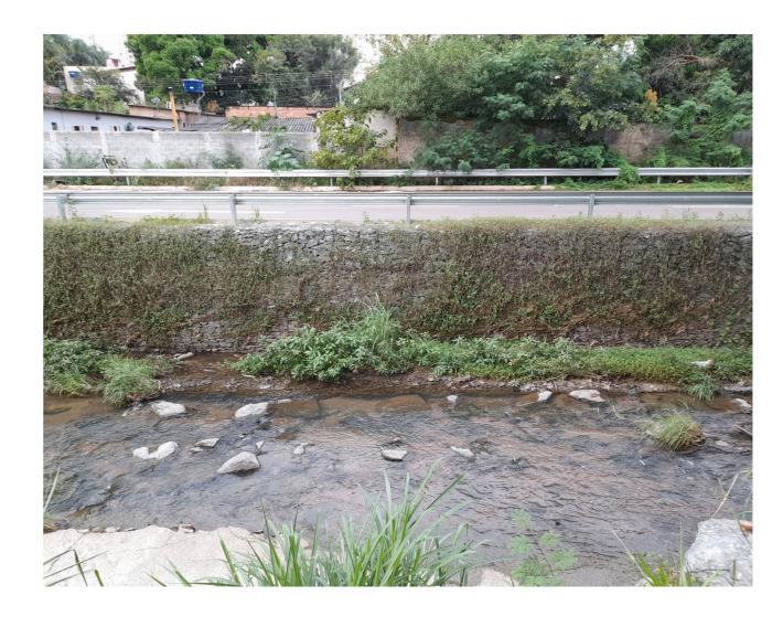
Figure 63 Gabion wall with spontaneous vegetation, Goiânia/GO (Collection of Belgo Soluções Geotech, photo: Flávio Fontes da Cruz, 2024).
