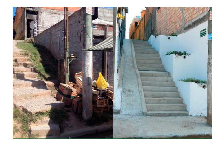
Figure 18 Vegetated hydraulic stairs in a project for the Grotas of Maceió/AL (Source: UN and Guajava, 2021).
